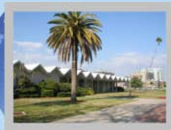
ICCE Davis Islands Facility
